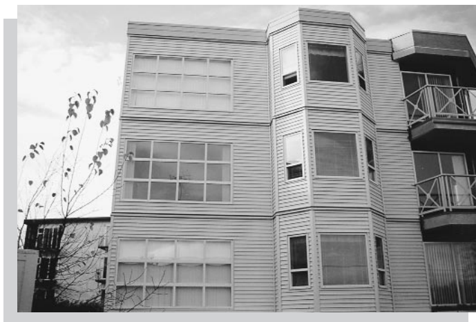
Completed Rain Screen Wall System
