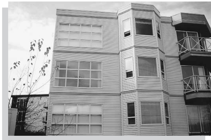
Completed Rain Screen Wall System
