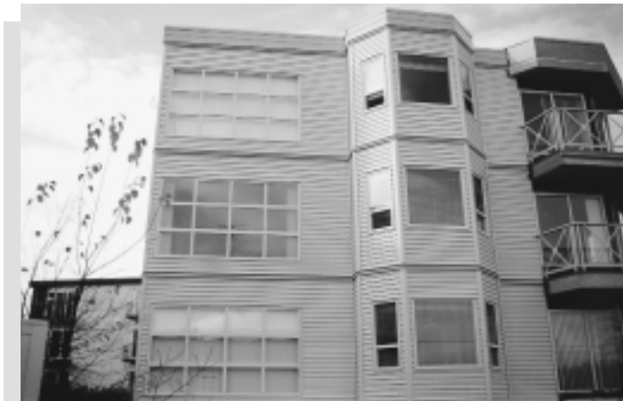
Completed Rain Screen Wall System
