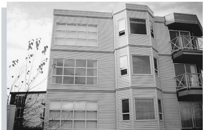
Completed Rain Screen Wall System
