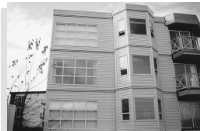
Completed Rain Screen Wall System
