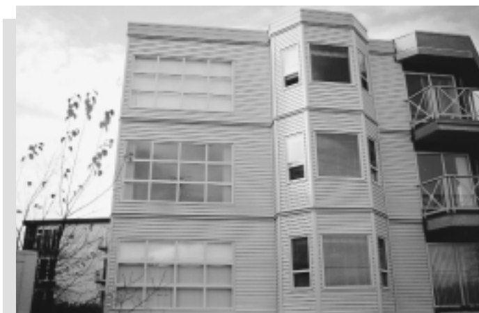
Completed Rain Screen Wall System
