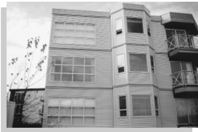
Completed Rain Screen Wall System
