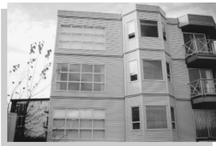
Completed Rain Screen Wall System
