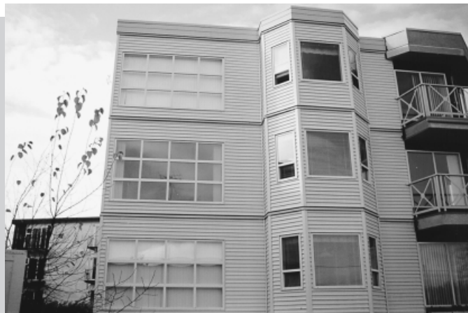
Completed Rain Screen Wall System
