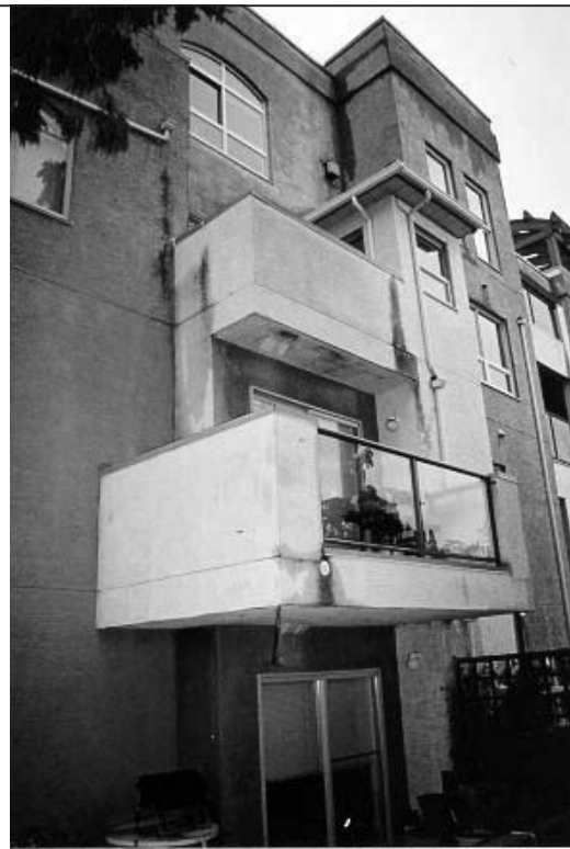
Before - clearly observable signs of systemic building envelope failure.
