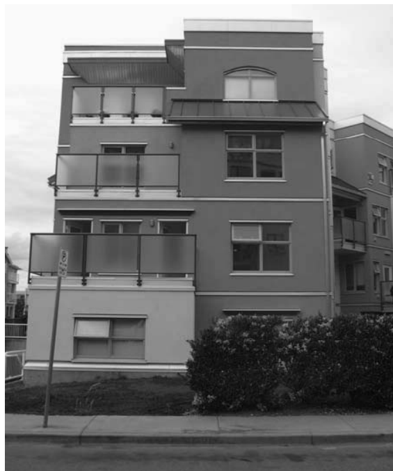
After - building envelope components repaired and/or replaced and properly installed in rain screen configuration. Note: balcony parapet walls removed and fascia mounted railings installed.
