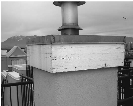
Weathered cedar trim – this state of weathering could have been prevented if maintenance was being carried out regularly after construction.
