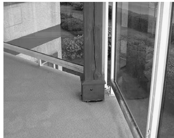
The deck membrane at the base of post is vulnerable to moisture ingress since it does not extend up onto the post. Also notice the splitting of the post.
